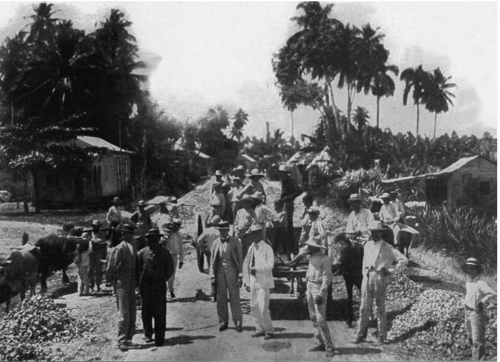
Foto 26 / "The Road near Aguadilla, Porto Rico"
